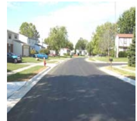
New pavement, curbs and gutters are in place on Lakefield Drive.
